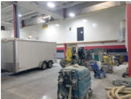
The MJA Company staging equipment for concrete polishing.
