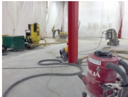
Floor preparation and polishing in progress. 2-shift production schedule.
